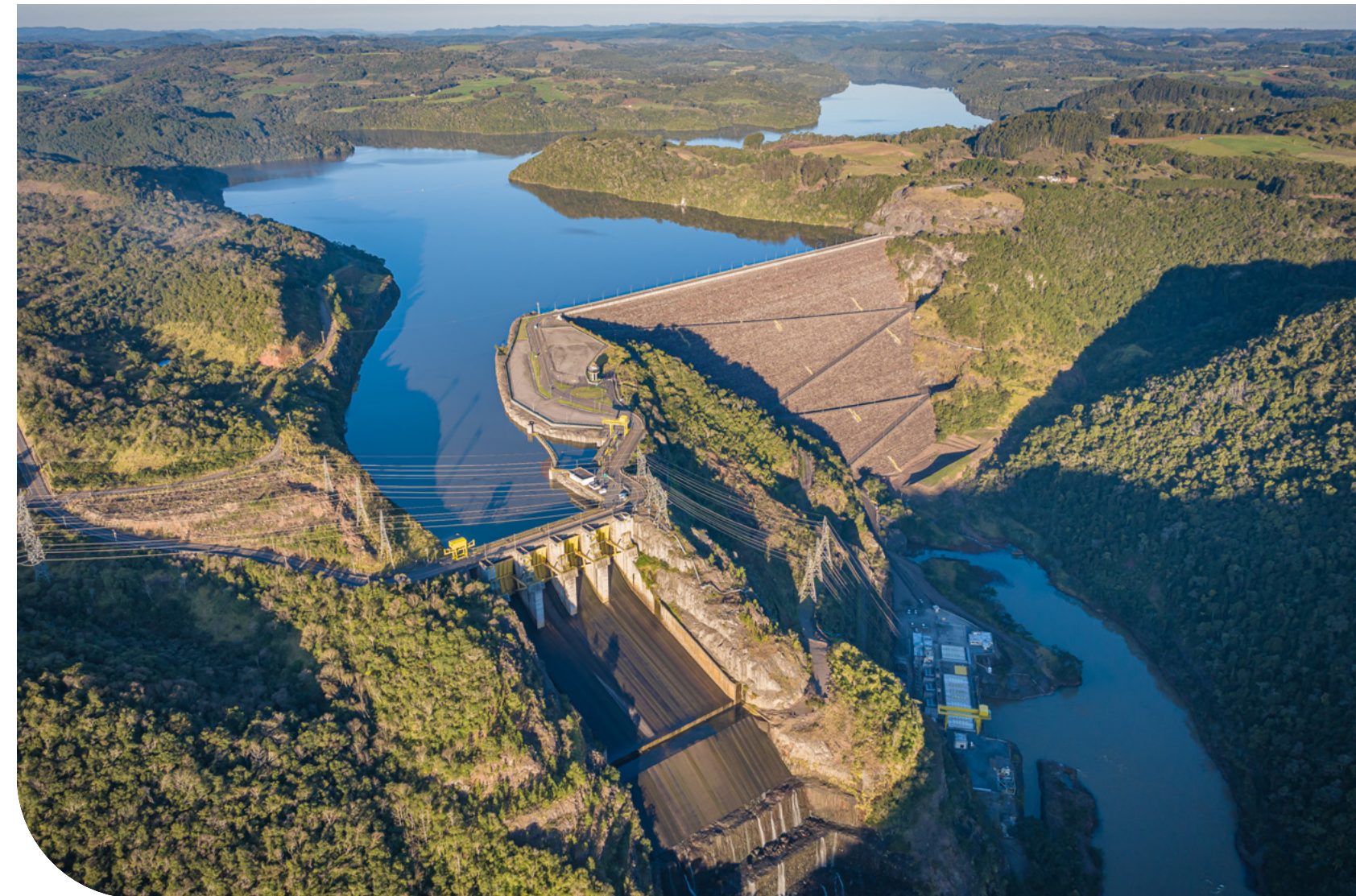
Campos Novos HPP Reservoir (Enercan), in Campos Novos (SC).
