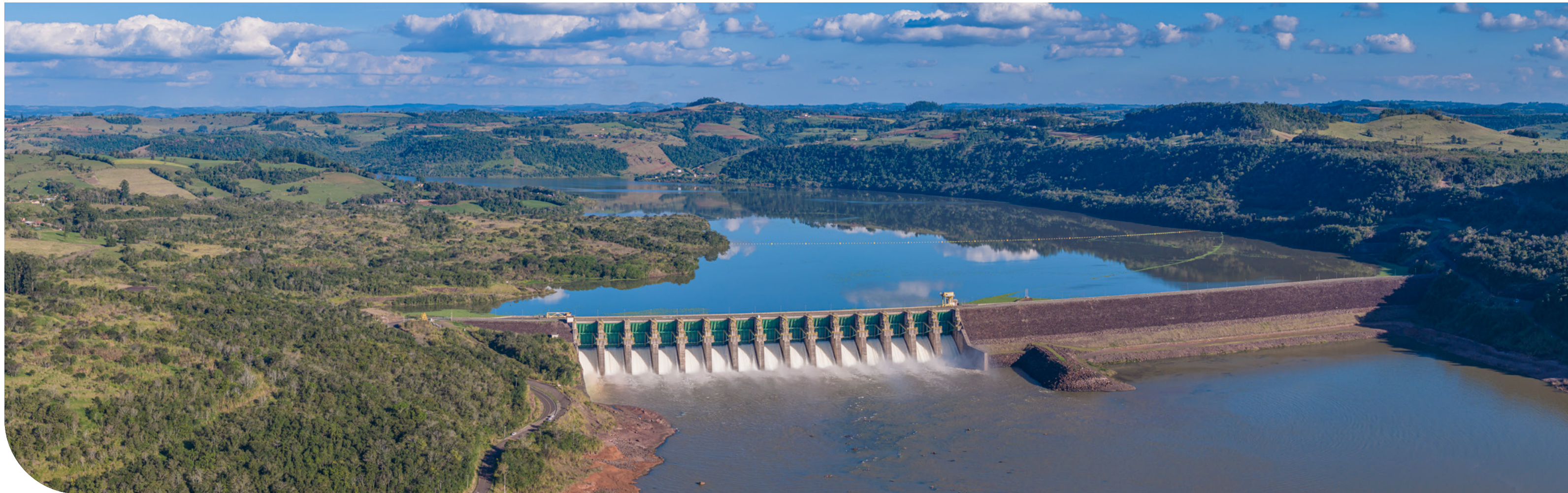
Foz do Chapecó hydroelectric plant, in Santa Catarina.
