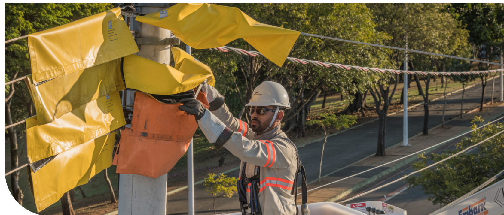
CPFL Piratininga network maintenance (SP).
