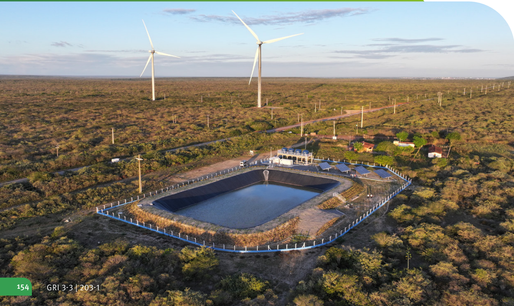
Water desalination plant built in the Rio Grande do Norte countryside.
