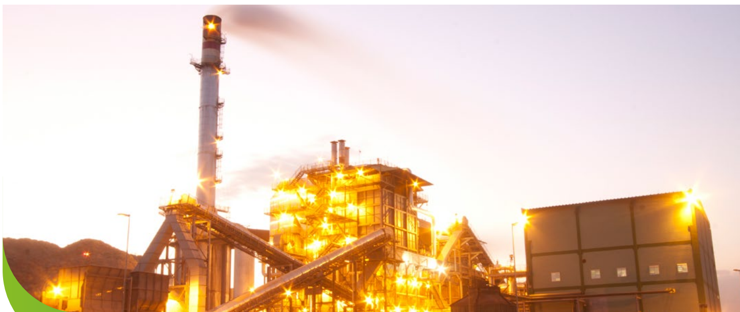
CPFL Renováveis biomass plant in Pirassununga - SP
