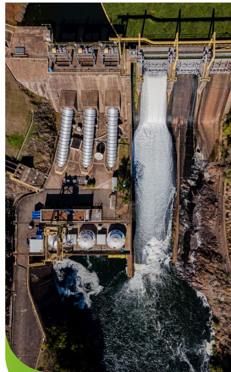
Small Hydroelectric Plant in Americana - SP
