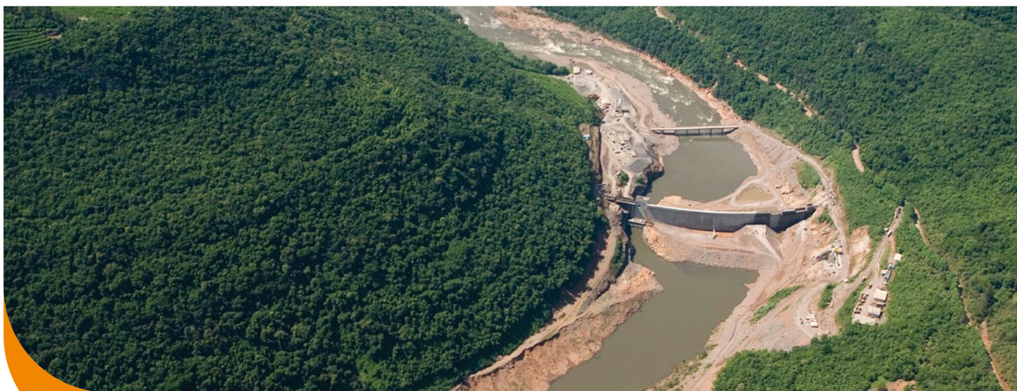
Castro Alves Hydroelectric Power Plant (Ceran)
