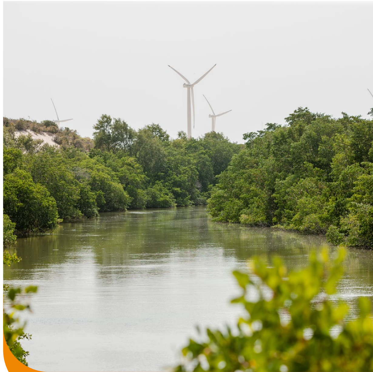
CPFL Renováveis Wind Power Plant in Ceará
