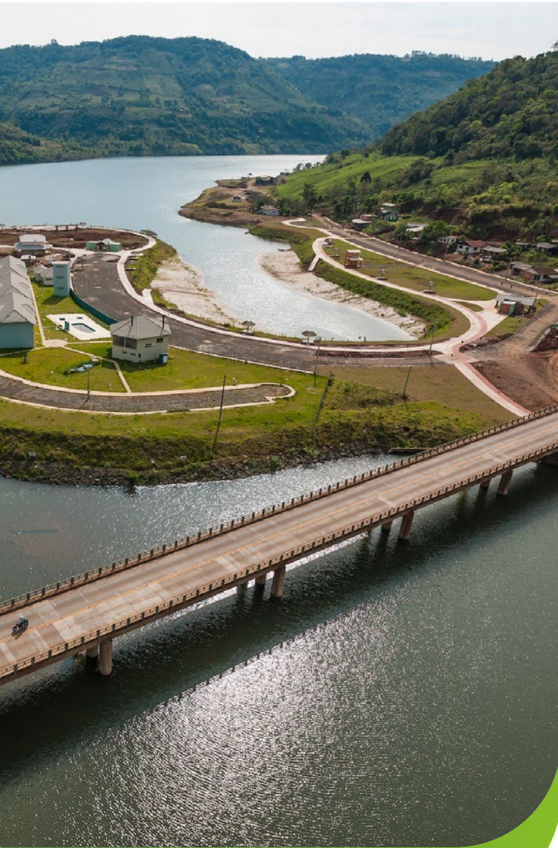
Foz de Chapecó Hydroelectric Power Plant
